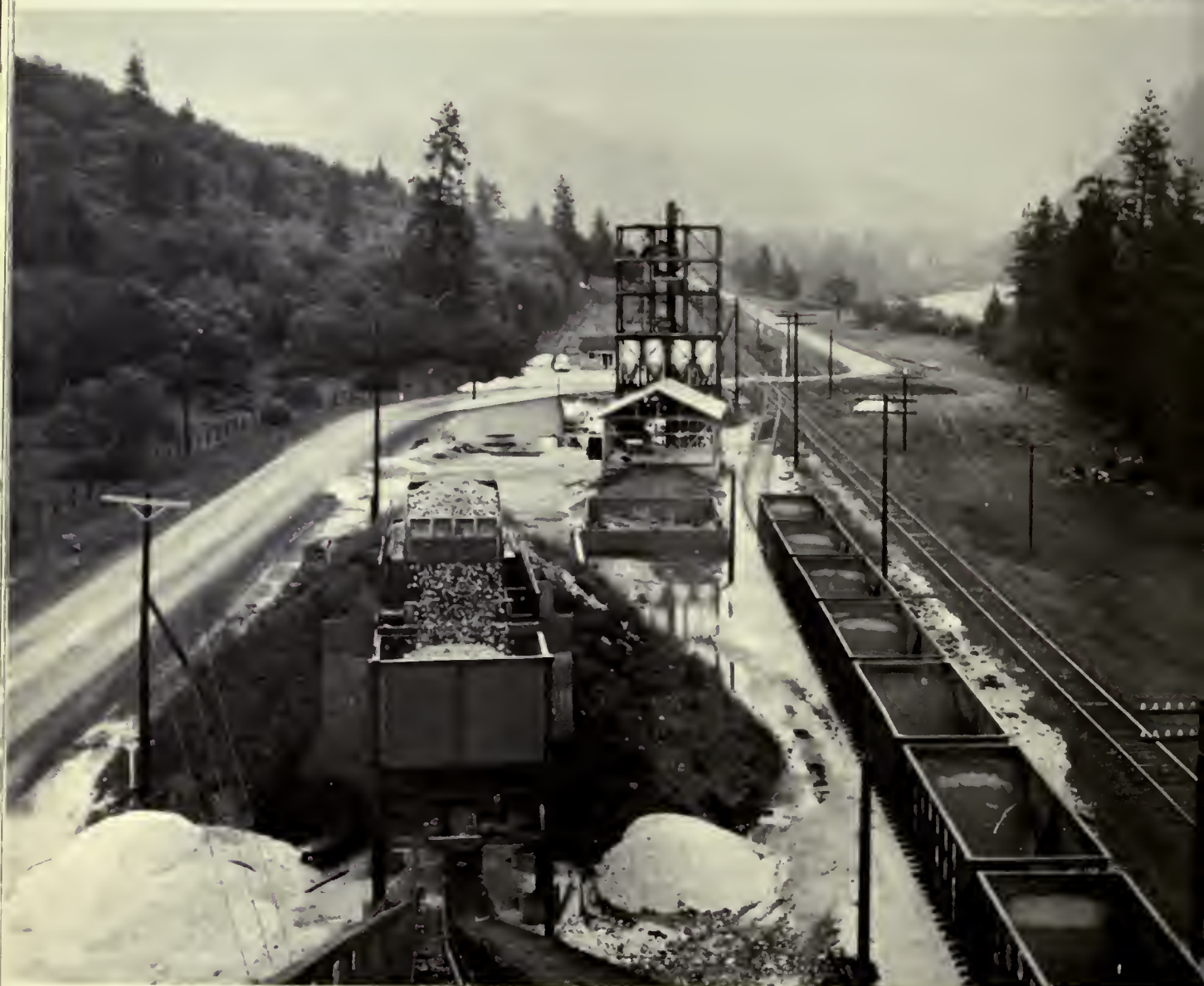
This plant near Gold Hill processes quartz into silica sand for industrial use in producing metals and glass.
